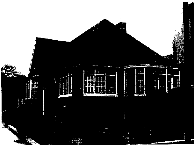
Figure 9: 7658 South Crandon Avenue
